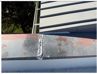
2. Added sealant between standing seam metal roof and parapet.
