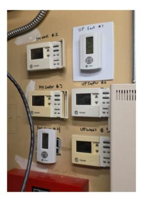
The sensors located throughout the building were non-adjustable and appeared to be averaging sensors to maintain a consistent temperature throughout the areas of the building that the rooftop is serving.
